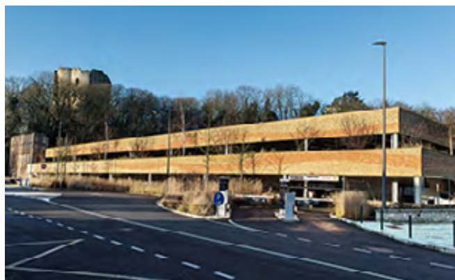
Insertion architecturale – Parking Relais de la gare d'Étampes (91)
